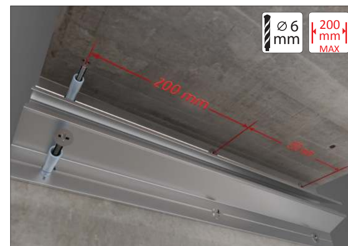
Fastening the profile to the concrete wall or ceiling
