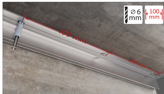
Fastening the profile to the concrete ceiling
