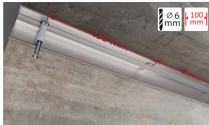
Fastening the profile to the concrete ceiling
